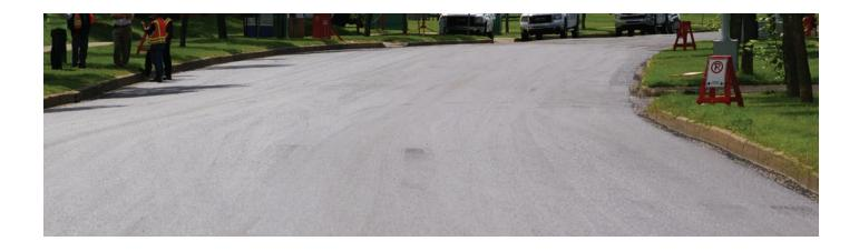
The cold aspect of EZ Street Asphalt allows for the paver joints to merge and bond together to form a single wide mat. For example a project with three paver runs will traditionally create two cold joints in the surface. Three paver runs with EZ Street Asphalt will leave no joints at all in the surface.
