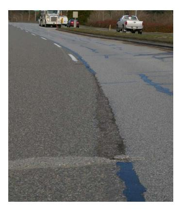
The one constant is that the joints will inevitably require maintenance expenditure over the life of the surface. In the worst case scenario, the full pavement may have to be resurfaced years earlier than programmed, causing significant adjustments to the programmed expenditure.
