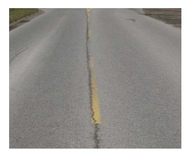
compression due to trafficking over these areas can lead to longitudinal cracking and general "alligator cracking". As soon as cold joint unravelling or cracking (longitudinal as well as alligator) occurs, the maintenance expenditures begin to climb.
