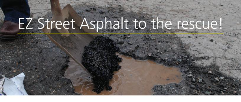
EZ Street is a high performance, polymer modified asphalt designed and produced with benefits exceeding that of regular asphalt but can be used with the same or better ease of cold mix.
