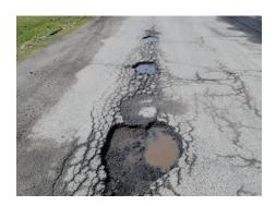
The most common repair material throughout the country is the utilisation of a standard cold mix or modified cold mix material. It is commonly known and experienced that these materials have a strike rate / permanency success rate of maybe 30%. This success rate percentage is up for debate around the industry and in many situations can be higher or significantly lower.
