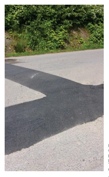
EZ Street is not subject to the normal "slabbing effect" commonly found when placing new asphalt to patch on top of existing asphalt.
